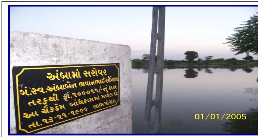
(D). Amba Sarowar, first check dam build near the Vikaliya village after Mrs. Ambaben donated 1, 00,011/- rupees for construction activity.
