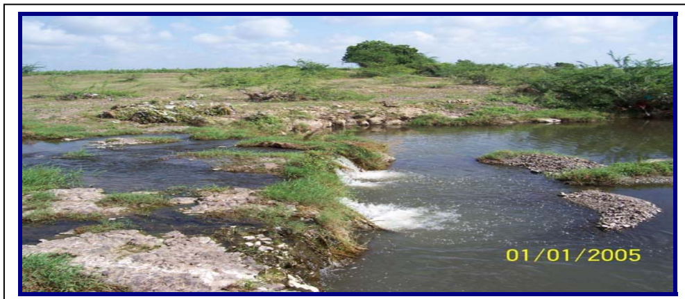
(E). Outlet of the sewage pipe lines.
