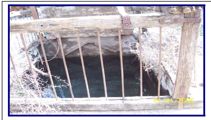
(C). Sewage outlet out side the village.
